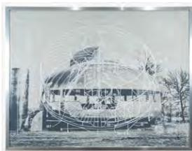
structure tensionally suspended from a central mast and braced to the ground. No single part weighed more than ten pounds or needed more than one hand to be held in place, making assembly feasible for one person. Most of the parts nested for shipping, and all the parts fit into a cylindrical shipping container. Cost estimates suggested that once the mass production phase was activated, the completed house, installed, could be sold for \$6,500.
